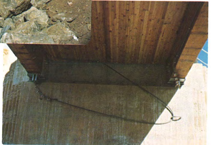
River embankment pier, showing cable which holds one section of the bridge to the bank of the river if flooding causes sections to float off the center pier.
