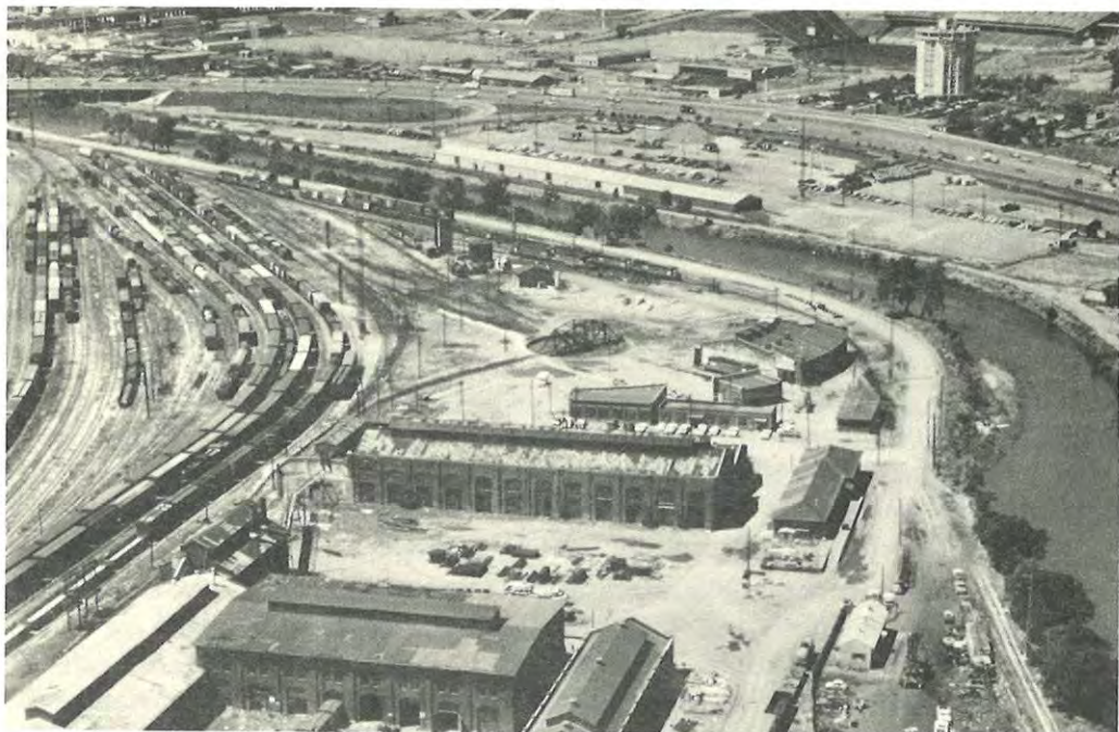
A part of railroad yards looking west across the river to Gates—Crescent Park (where the Children's Museum will be located). Mile High Stadium and McNichols Arena are in background.
