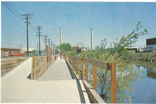
Same section of river after cantilevered deck was built between railroad track and river.
