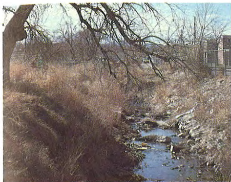
Weir Gulch, north of 8th Avenue, before improvements.
