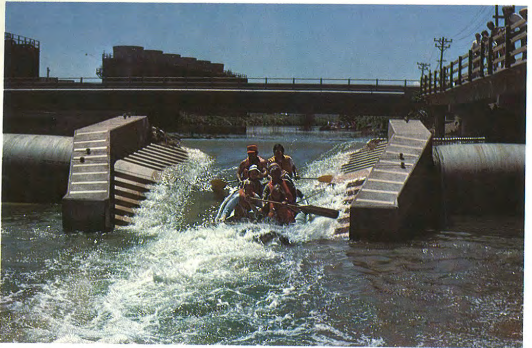
Zuni boat chute, resting on Public Service Company's fabri-dam at 13th Avenue.
