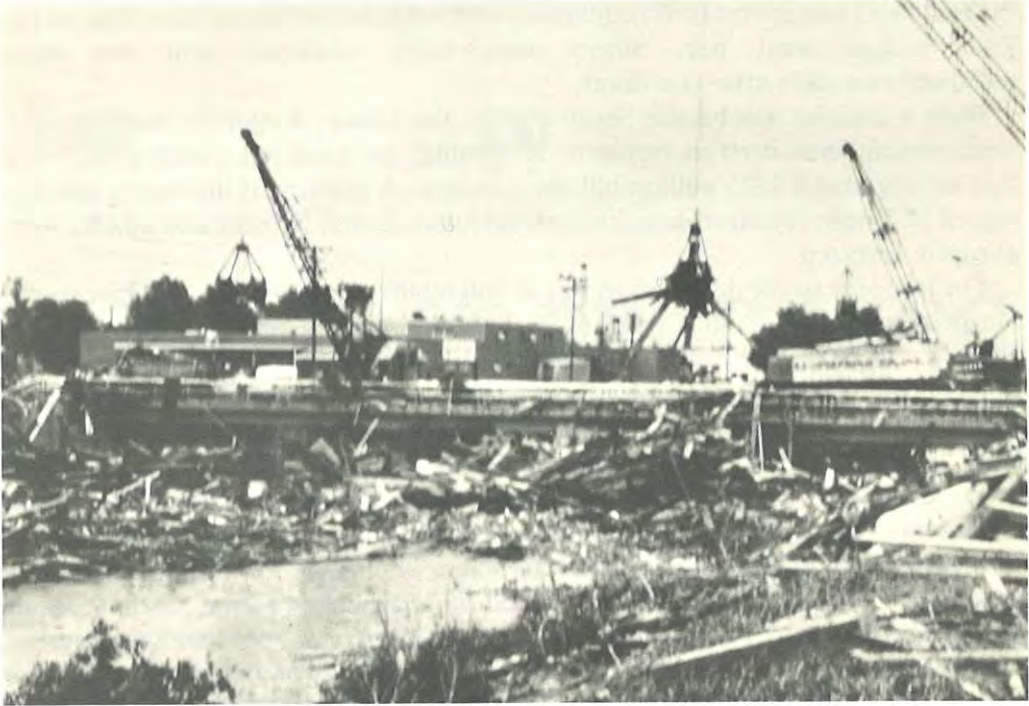
1965 flood aftermath, showing debris clogging the 8th Avenue bridge.
