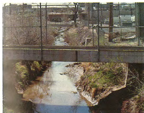
Lakewood Gulch, looking west from the river, as it appeared before the Committee went to work.
