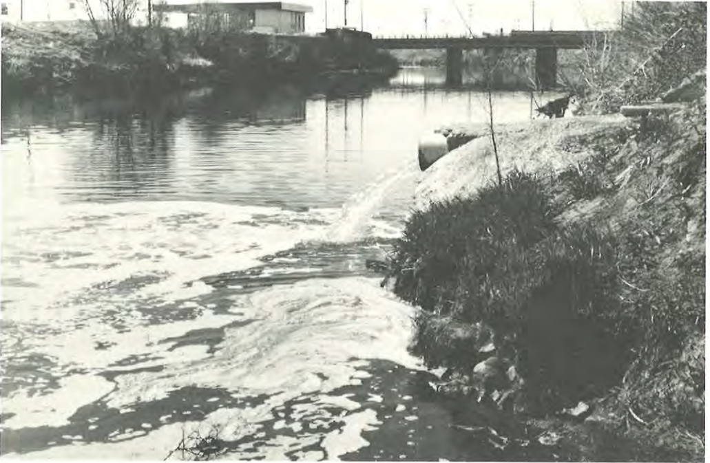
The discharge by local treatment plants, such as this by Lakewood Sanitation District at 9th Avenue, requires constant monitoring and testing to upgrade water quality.
