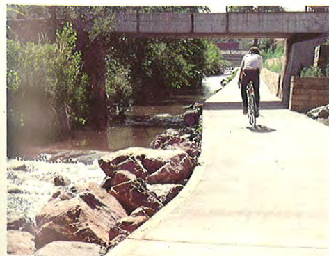
Lakewood Gulch, with hike-bike trail of warm-tone concrete, flood resistant, after development.
